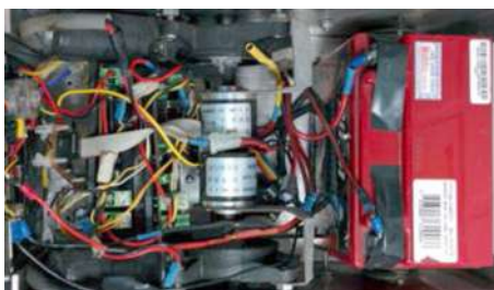
Figure 16. Electrical system: motor drivers, encoders, DC motors, shunt board and the 12V battery.
